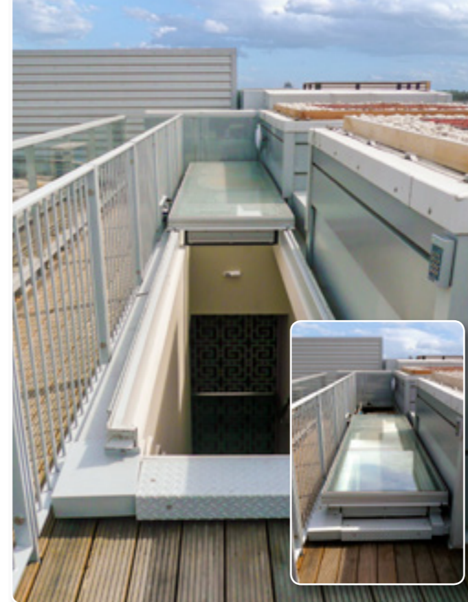
Sliding Glass Roof Access - London
